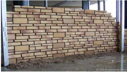
Figure 1: An example of a polymetric brick wall from [www.metselen.net/fotoalbum.html](http://www.metselen.net/fotoalbum.html)
